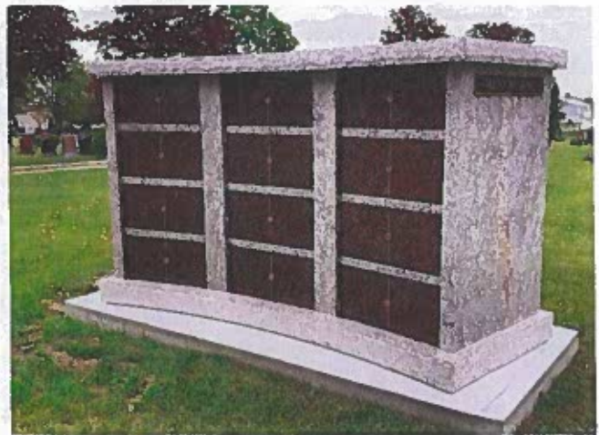
Figure 6: 48 Niche Curved Columbarium Arctic Grey with Canadian Mahogany Doors, Eden Church Cemetery, Cambray, ON
