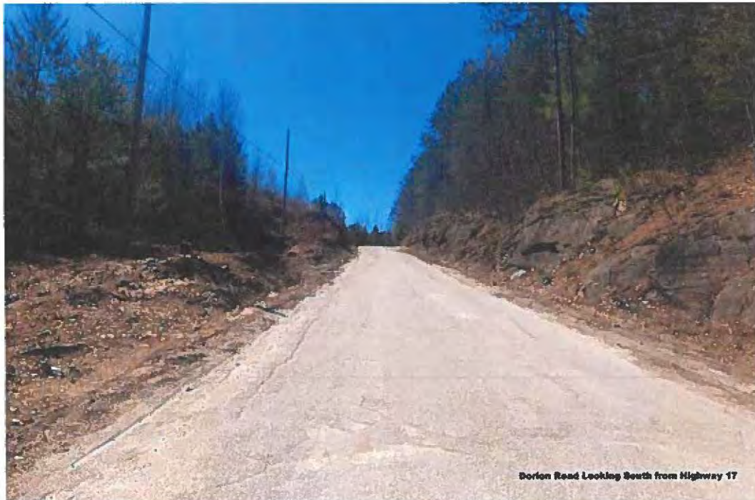
Figure 2A Dorion Road Hill looking South to “new curve”
