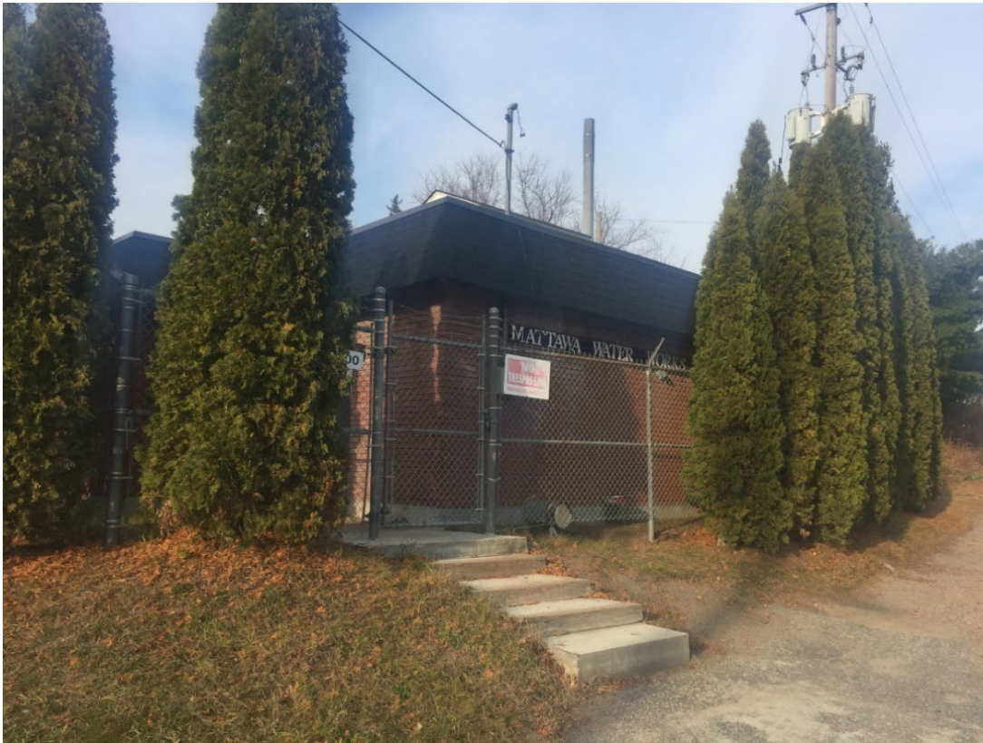
Figure 12 Photo of Existing Water Treatment Plant
