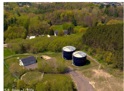
Ground Level Storage Facility
