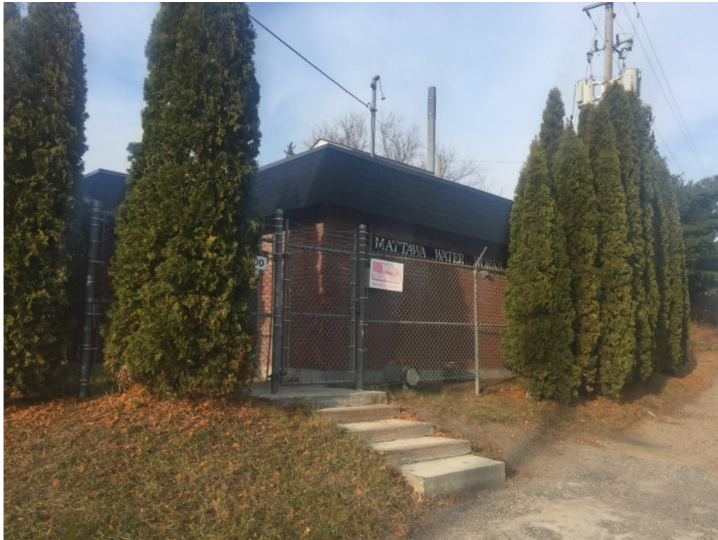
PHOTO 11 TOWN OF MATTAWA WATER TREATMENT PLANT
