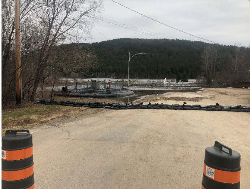
PHOTO 4 BROOK STREET DURING MAY 2019 FLOOD
