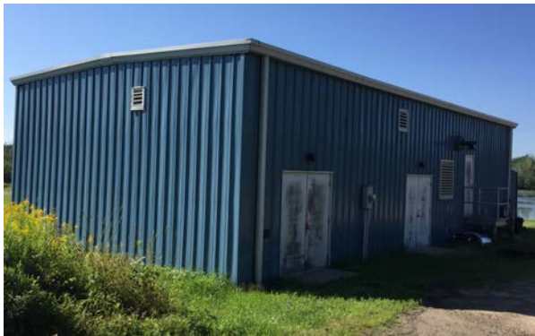
PHOTO 14 TOWN OF MATTAWA SEWAGE TREATMENT PLANT (BLOWER BUILDING)
