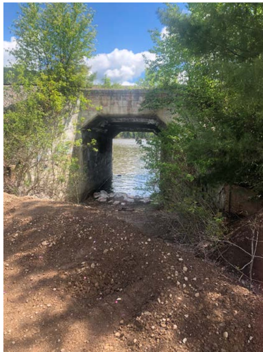
PHOTO 10 CPR BOX CULVERT AT TIMMINS STREET
