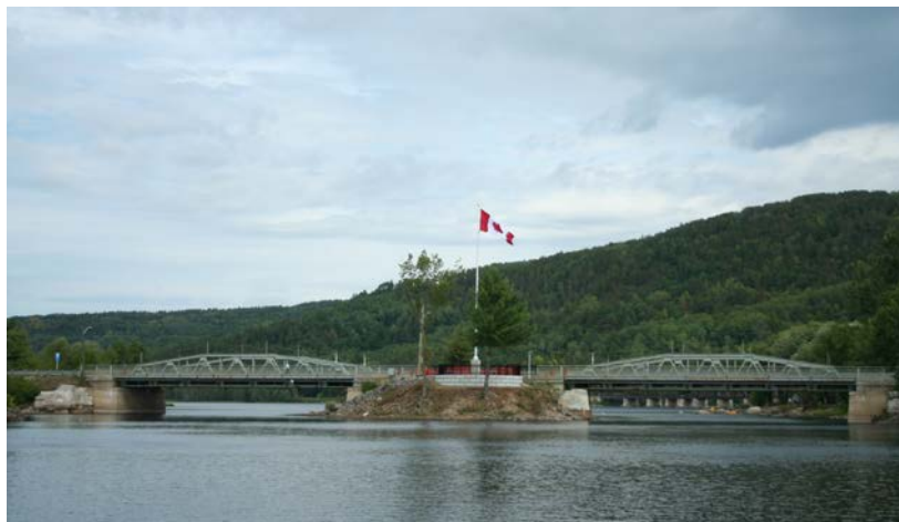
PHOTO 5 MAURIL BÉLANGER BRIDGE
