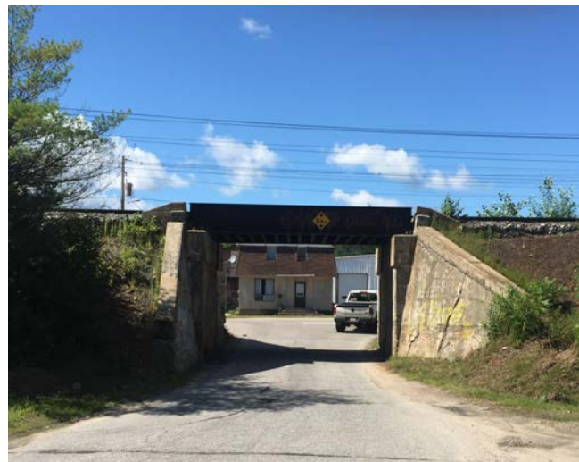
PHOTO 7 CPR/DONALD STREET OVERPASS
