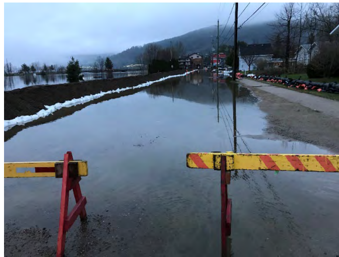
FIGURE 27 PHOTO MATTAWAN STREET DURING MAY 2019 FLOOD
