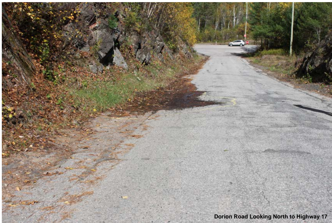
Figure 2B Dorion Road Hill looking North to Highway 17 Intersection
